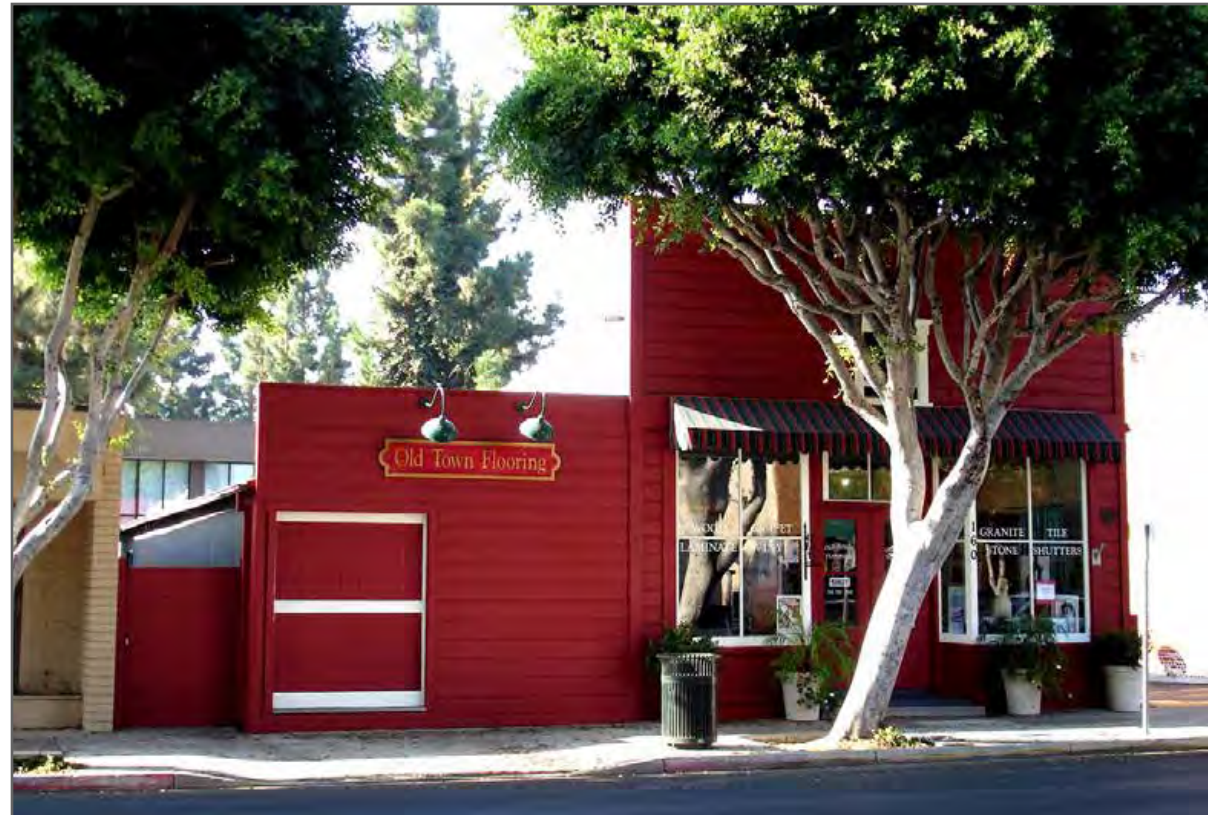
Old Town Flooring – McCoy's Sheet Metal Building at 160 East Main Street
