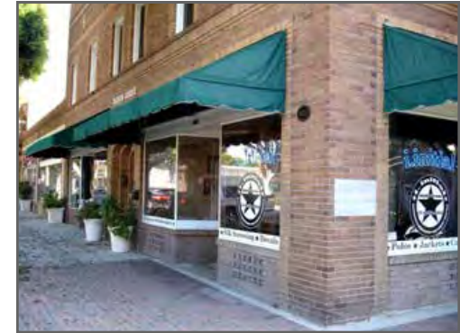
Awning on Knights of Pythias Building at 397-399 El Camino Real.
