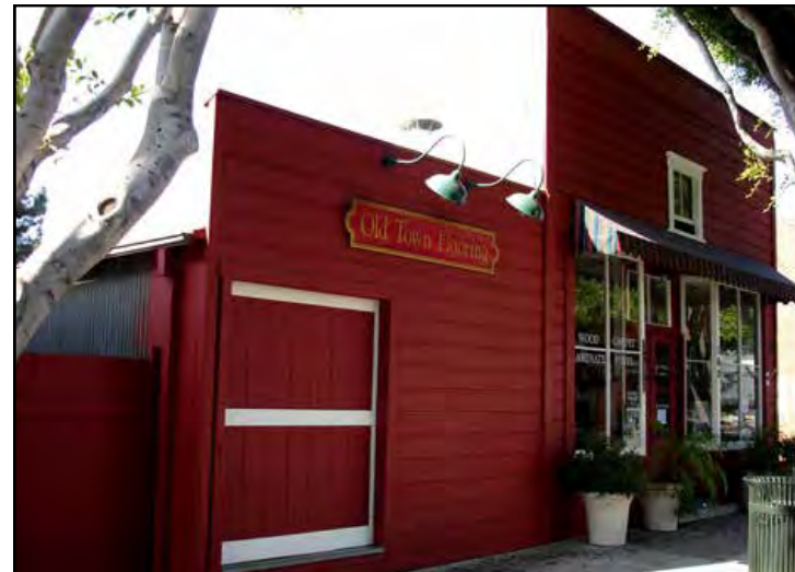
8. Old Town Flooring – McCoy's Sheet Metal Building
