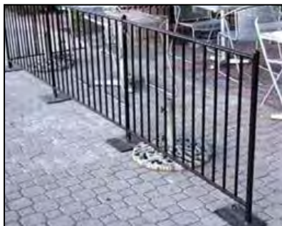
Sectional fencing in the form of railing with a stanchion base of no more than 1/2 inch helps minimize the hazard of tripping for patrons and other pedestrians.
