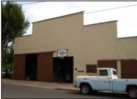
Blacksmith Shop at 245 South C Street.
