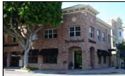
191 East Main Street (Commercial Building)
