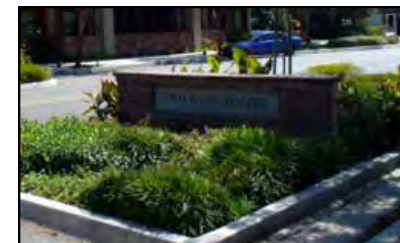
Bioretention planter with a monument sign provides a barrier between traffic and pedestrians along El Camino Real.
