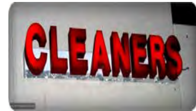
Lighting does not fit lettering properly. Neon signs are discouraged.
