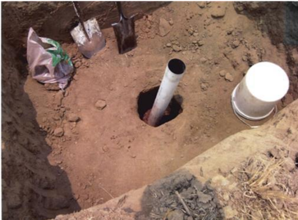
Figure VII.17. Photo of Percolation Test Pit.
