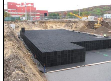
Underground detention tank Source: www.webtecgeos.com
